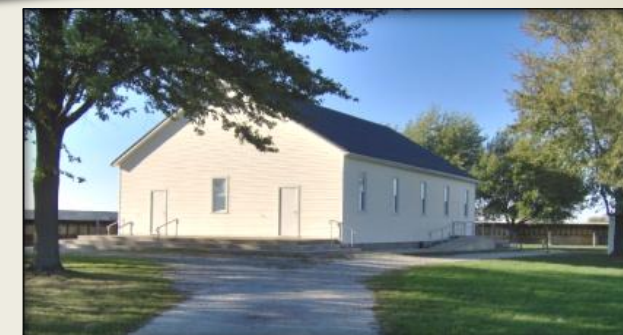
Clearland reconstructed church from lumber that had already served 99 years as a church.
